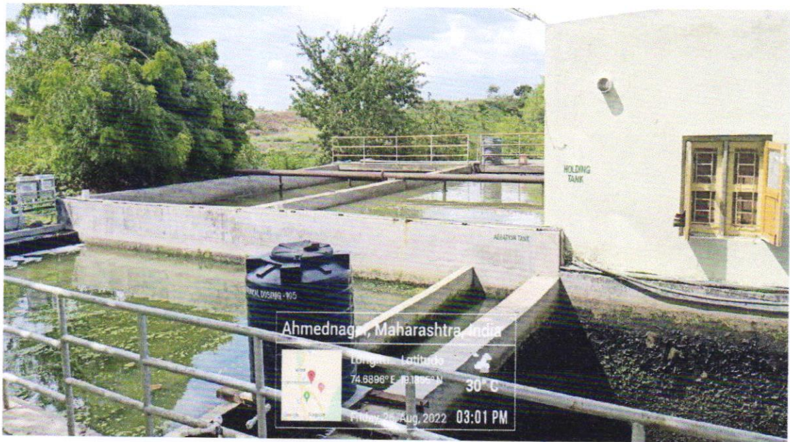
Aeration Tank and Holding Tank
